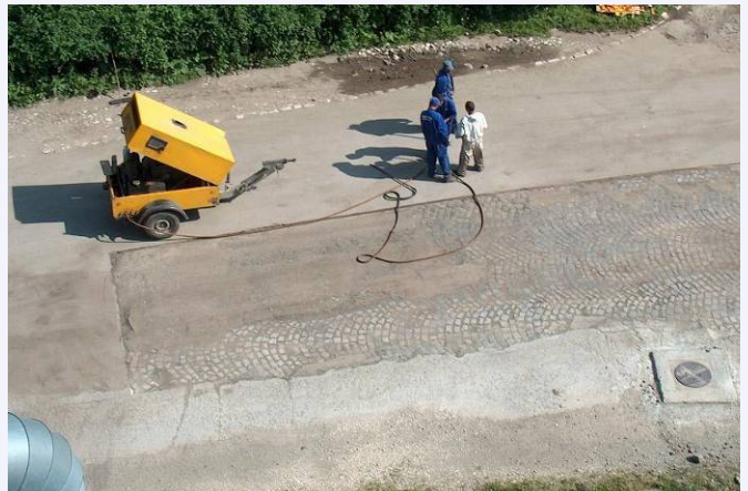
Frezarea zonelor puternic deteriorate
